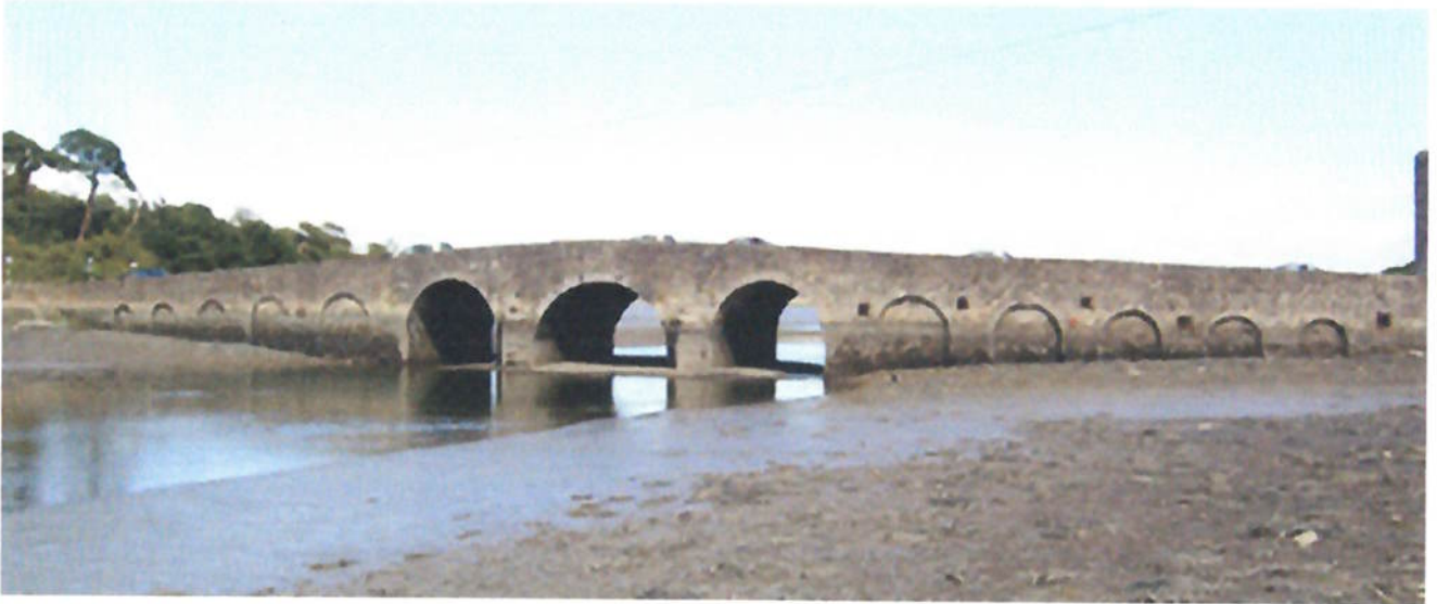
Belvelly Bridge, BELVELLY, CORK - Buildings of Ireland
